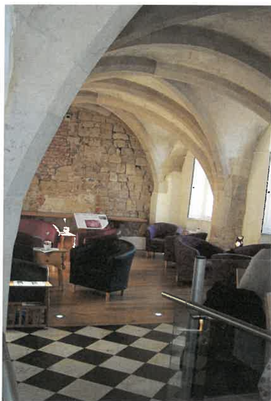
Groyne vaulted ceiling in Priory House
