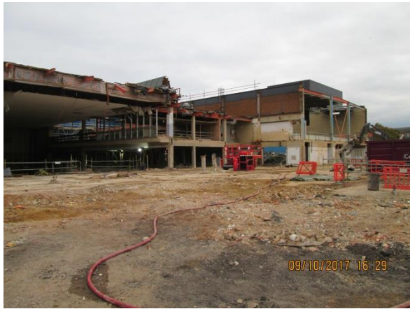
Demolition Complete to Pool and Sports Hall
