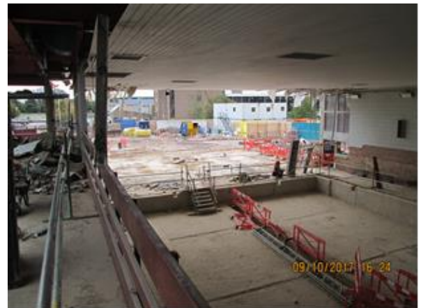
Swimming Pool East Wall Removed
